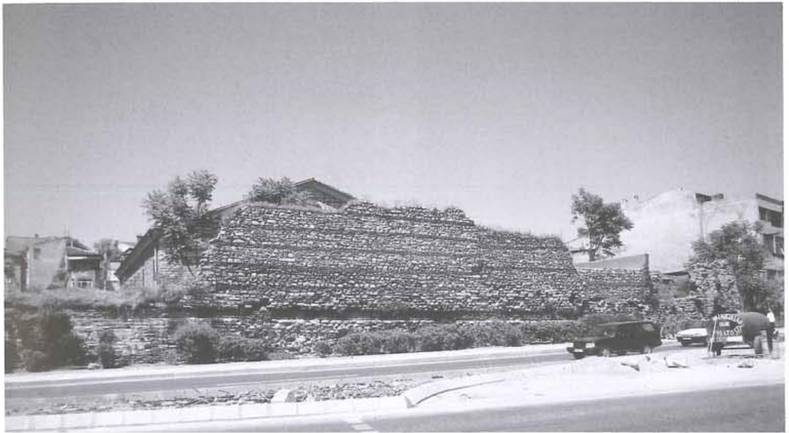
Plate 67 Walls along the Golden Horn
